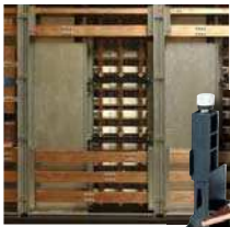
SB P 10: 1 bar with a thickness of 5 or 10 mm, width 12, 20, 25 or 30 mm.
