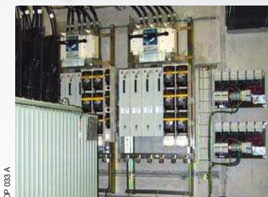
DIN type switchboard (for TN earthing system distribution)
