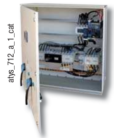
Steel enclosure with changeover switches
