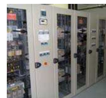
Pre-cabled distribution board
